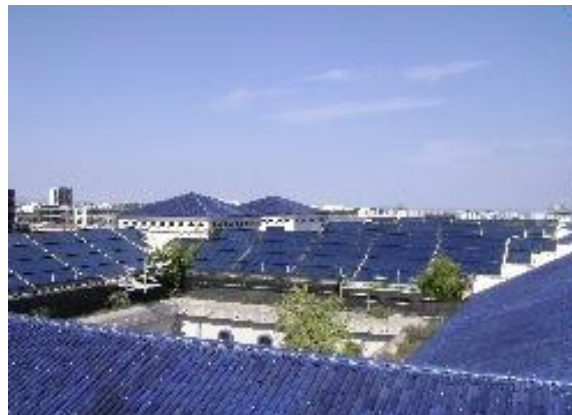
CGD, Portugal. Large flat plates, absorption, 545 kW.
