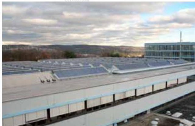
Festo, Germany. Evacuated tubes, adsorption, 1050 kW.
