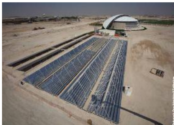
Stadium, Qatar. Linear Fresnel, absorption 2-effect, 750 kW.
