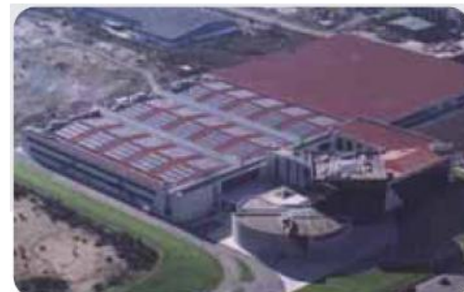
Inditex, Spain. Flat plates, absorption, 150 kW.
