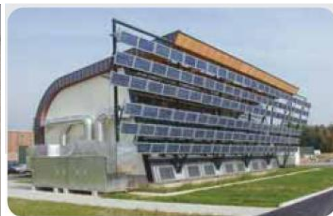
Ökopark Hartberg, Austria. Flat plates, dessication, 30 kW.
