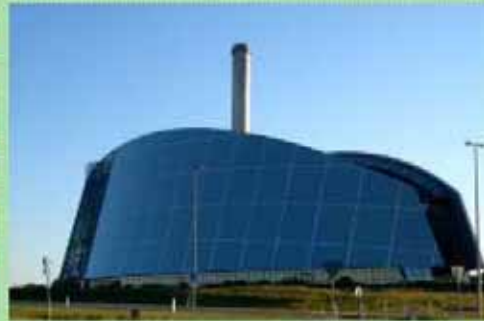
The New incinerator power plant
